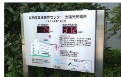
Sign showing output from the solar power system
