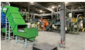
Our facilities to crush and select roasted batteries
